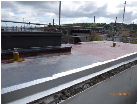
Looking West: Man safe roof brackets and cable restraint insitu.
