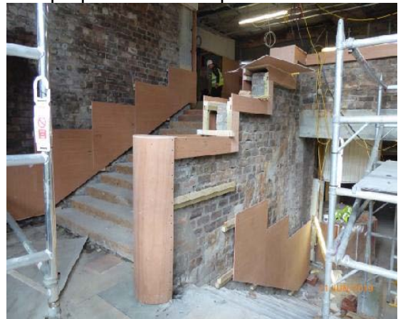
General view of Main Staircase (Half-Landing) – plywood template sheeting now fitted for the new wall paneling.
