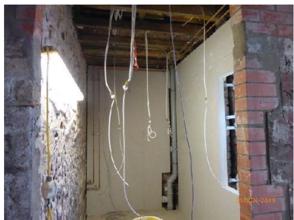
Ground Floor: New Accessible WC.
