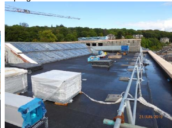
Looking North: General view East area adjacent Argyle Street.
