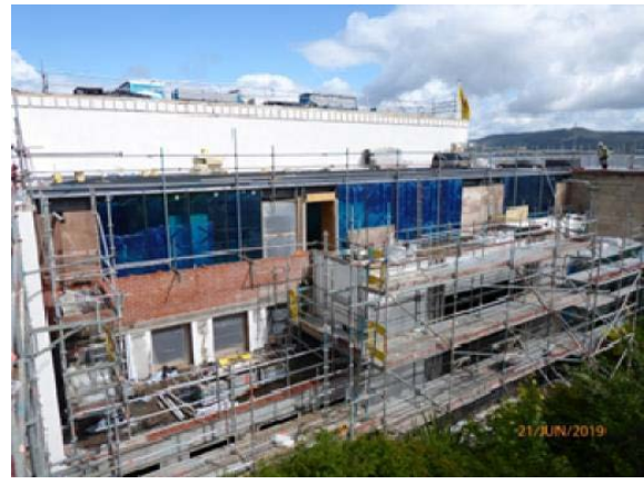
South Elevation – General view.
