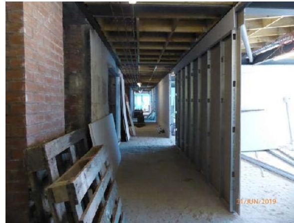
New Offices: General view of Corridor looking East.
