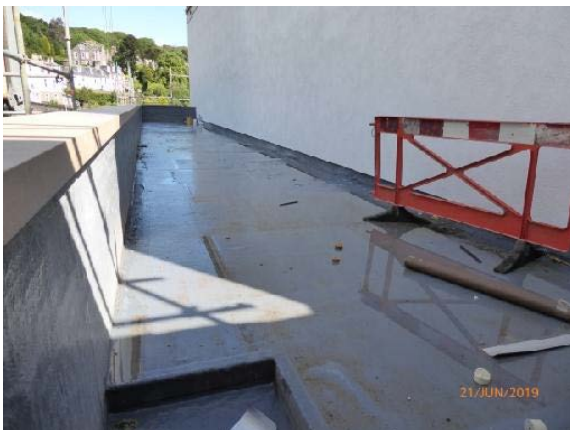
Looking North: West Elevation: First floor – General view.
