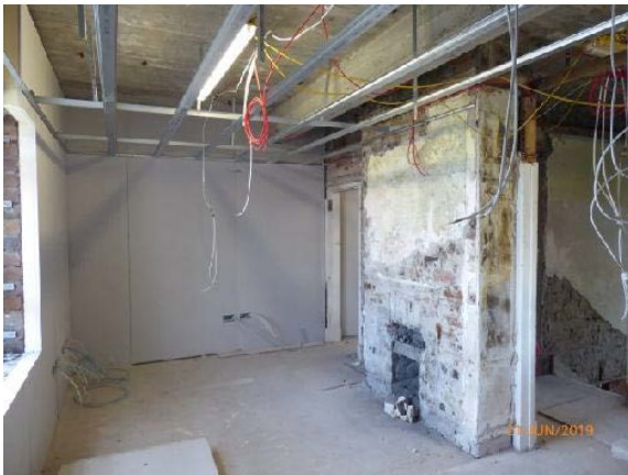
First Floor: General View of new Office
