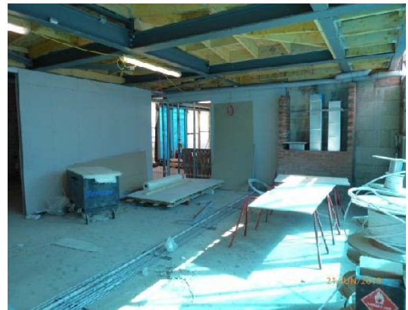
New Office adjacent Staircase 1 (South Elevation – looking East): Brickwork to new service riser visible.
