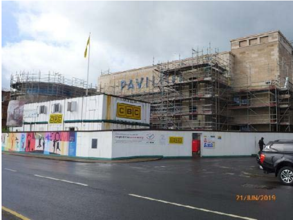
East Elevation (Argyle St.) – Front Elevation (NB: new PAVILION sign insitu).
