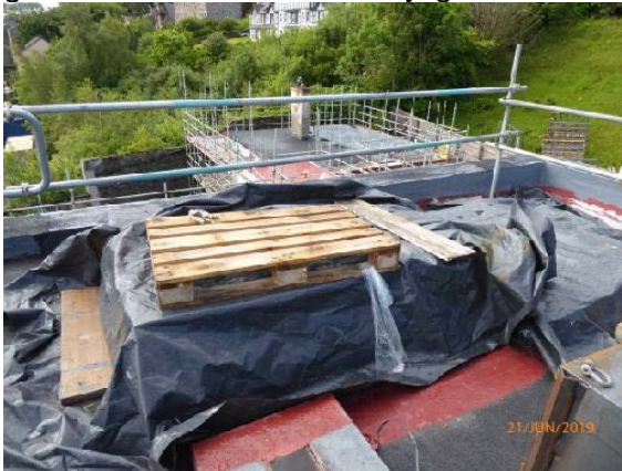
Looking SW: General View – roof finishes awaiting completion south west corner...
