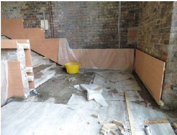
General view of Main Staircase (Half-Landing) – plywood template sheeting now fitted for the new wall paneling.
