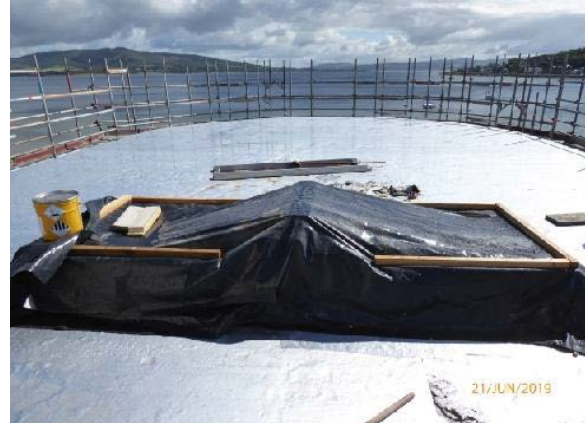
Looking East: General View of the roof over the Exhibition/Function Suite.
