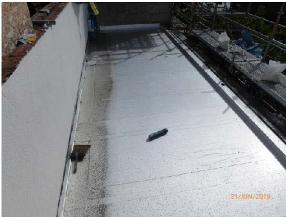
General views: Roof over Shop.
