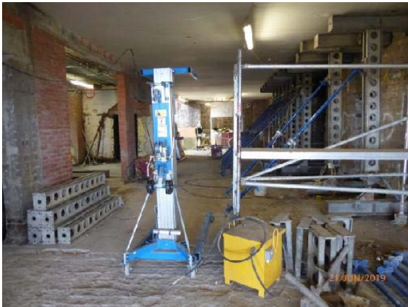
Looking West: (towards box office): General view of Main Entrance Foyer/Circulation area.
