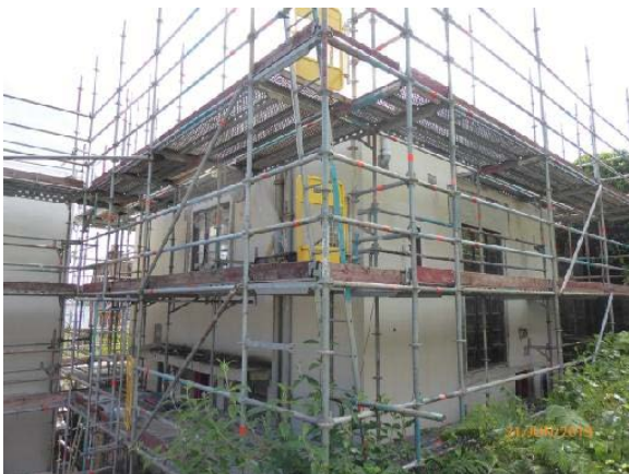
West & South Elevations – Caretakers House (NB: new windows in situ).
