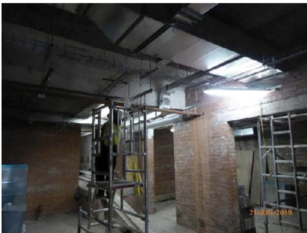
Male WC – Electrical wiring in progress.
