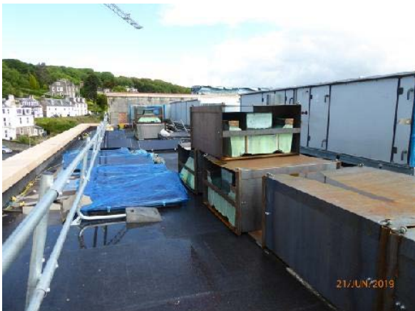
Looking North: General view west area.
