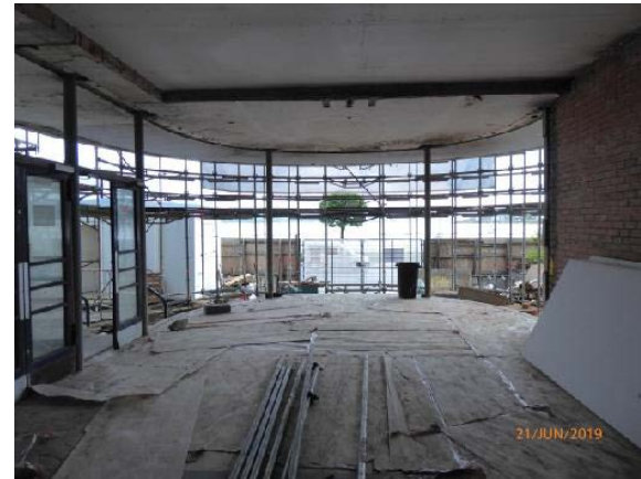
Looking East (Argyle Street): General view of Entrance Lobby.
