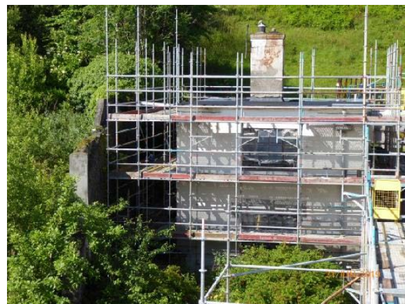
East Elevation – Caretakers House.
