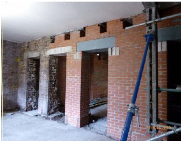
Looking West: New Female & Male WC door openings now substantially completed.
