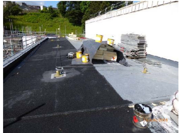
Looking West: General view of new roof over first floor offices. NB: Man safe roof brackets and cable restraint system insitu.
