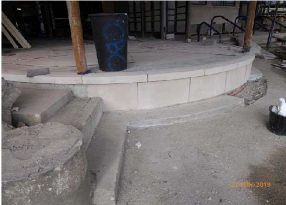
Main Entrance Lobby (facing Argyle St. - new cast stonework.
