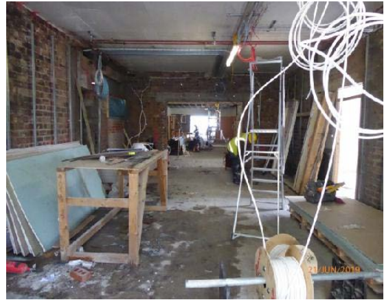
Looking East: General view of Multipurpose Flexible space area.
